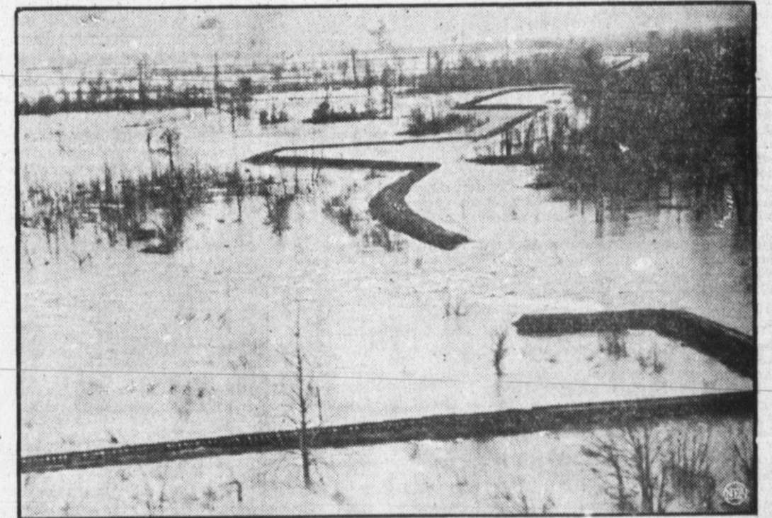
Ravaged by previous disastrous floods, the section around Kennett, in the extreme southeastern part of Missouri, again was swept by a deluge, the scene above showing a great gap torn in the levee by the surging waters of St. Francis river. In the foreground is a railway line, barely above the torrents, and a great stretch of fertile farmland was submerged. Hundreds of lowland residents were driven from their homes and more than 2000 refugees were cared for in Kennett, a city of 2500 population, by relief agencies.
