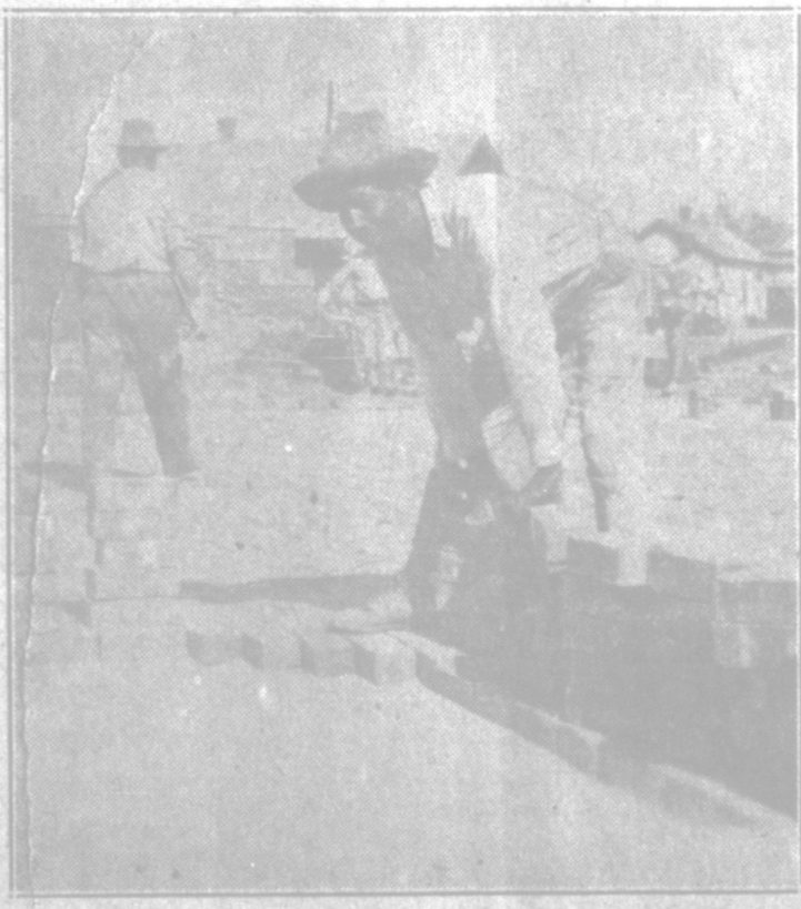
L. J. "Indian Jim" Brown, world's champion bricklayer, quickly and efficiently covered the concrete base on Pampa's wide streets. He was very interesting to watch.
