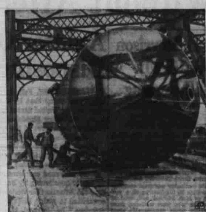
BRIDGE PROBLEM—Steady hands and quick footwork were needed by the men who helped roll this chemical storage tank across a bridge between Lackawanna, N. Y., and Niagara Falls, N. Y. The tank, 15 feet in diameter, was too high on a truck.
