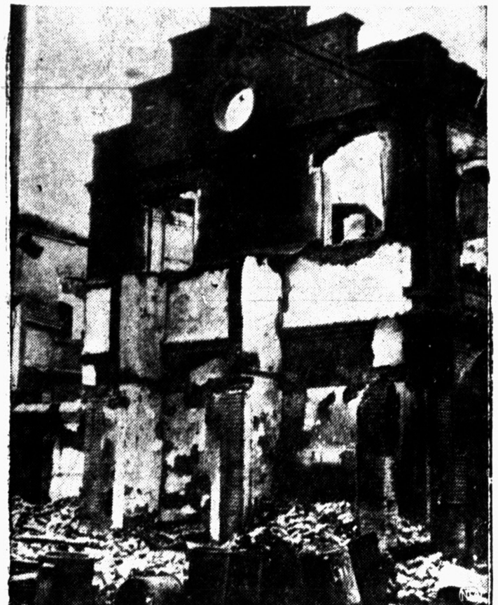
Japanese forces have spared neither lives nor property in their determined drive to gain control of North China. Many blocks of buildings in the path of the conquering army look like this: shell-shattered, smoke blackened skeleton in Tientsin
