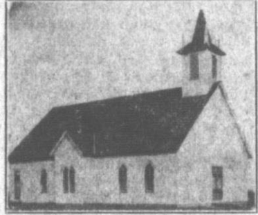
The new building will be the scene of an "open house" social gathering Friday evening for members of the church and their friends. There will be a brief program, and refreshments will be served by members of the church.
