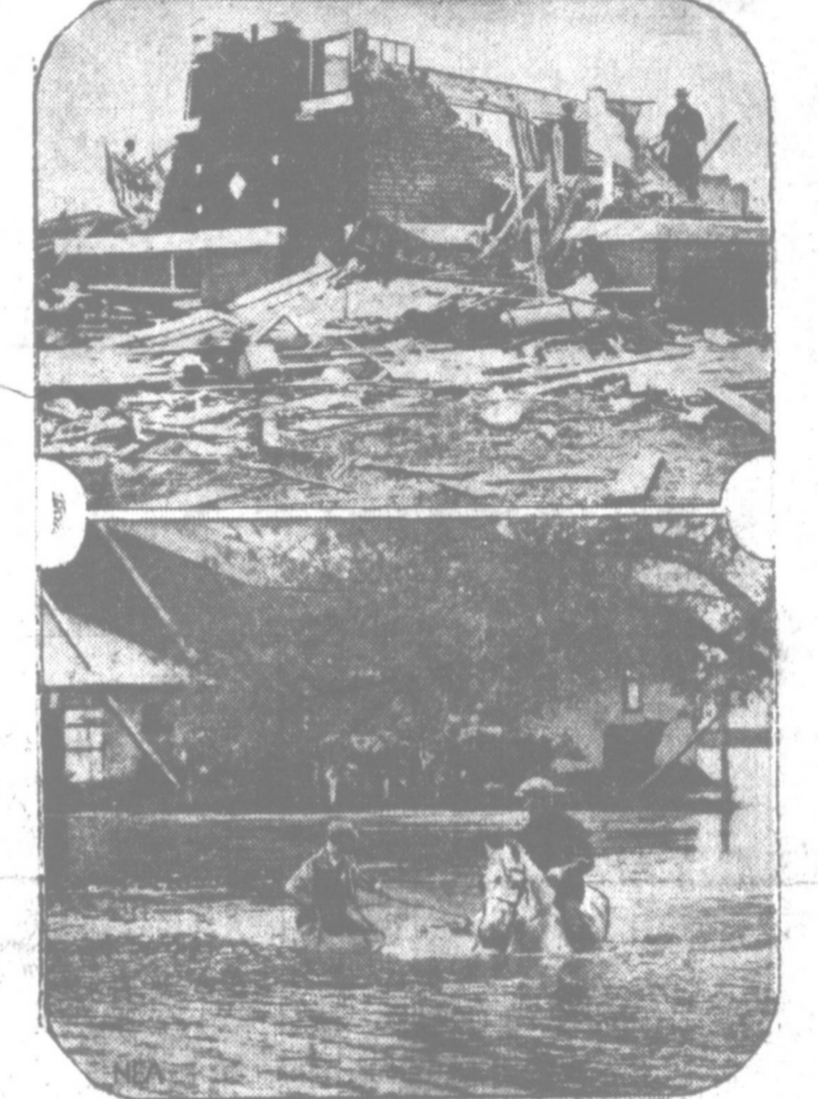
Missouri and Kansas have been hard hit by tornadoes and heavy rains which caused rivers to rise out of their banks, causing thousands of dollars in damages. The picture above illustrates the severity of the storms at Bolivar, Mo. The owner of the home suffered a broken back. Below, floods in the Kaw Valley near Menoken, Kas., are shown. The two boys on horseback have just carried feed to the cows on the elevation in the background.
