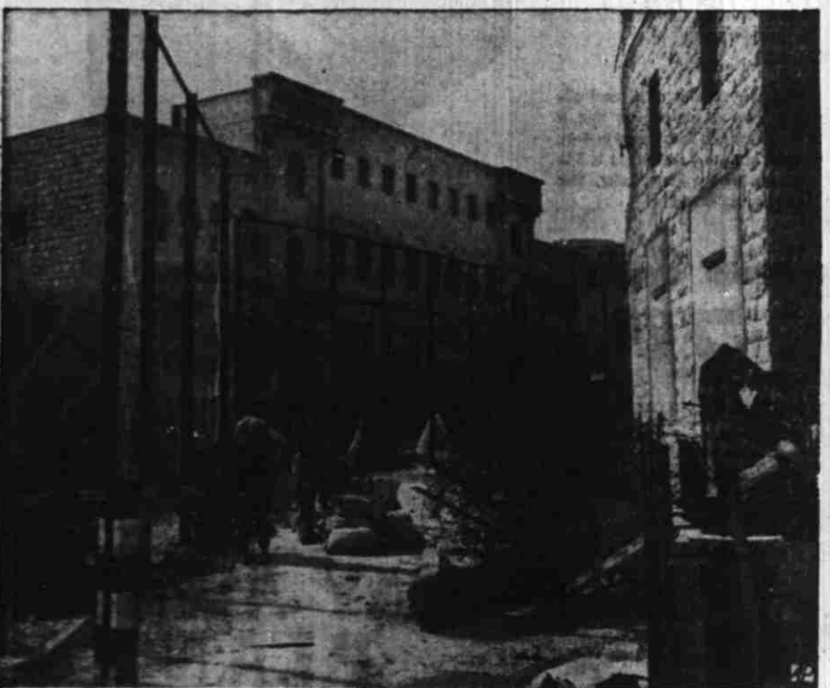
ANTI-TERRORIST FENCE — Wire netting is stretched between steel poles to protect Jerusalem headquarters of the Palestine police against possible terrorist attacks.
