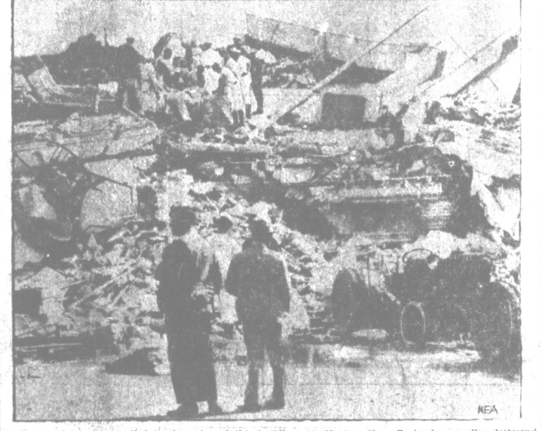
At least a dozen nurses died in the ruins of this building at Napier, New Zealand, recently destroyed by an earthquake. Sailors are seen digging in the debris for bodies. The tangled wreckage of this demolished nurses' home is typical of the ruin which killed scores and left many homeless.
