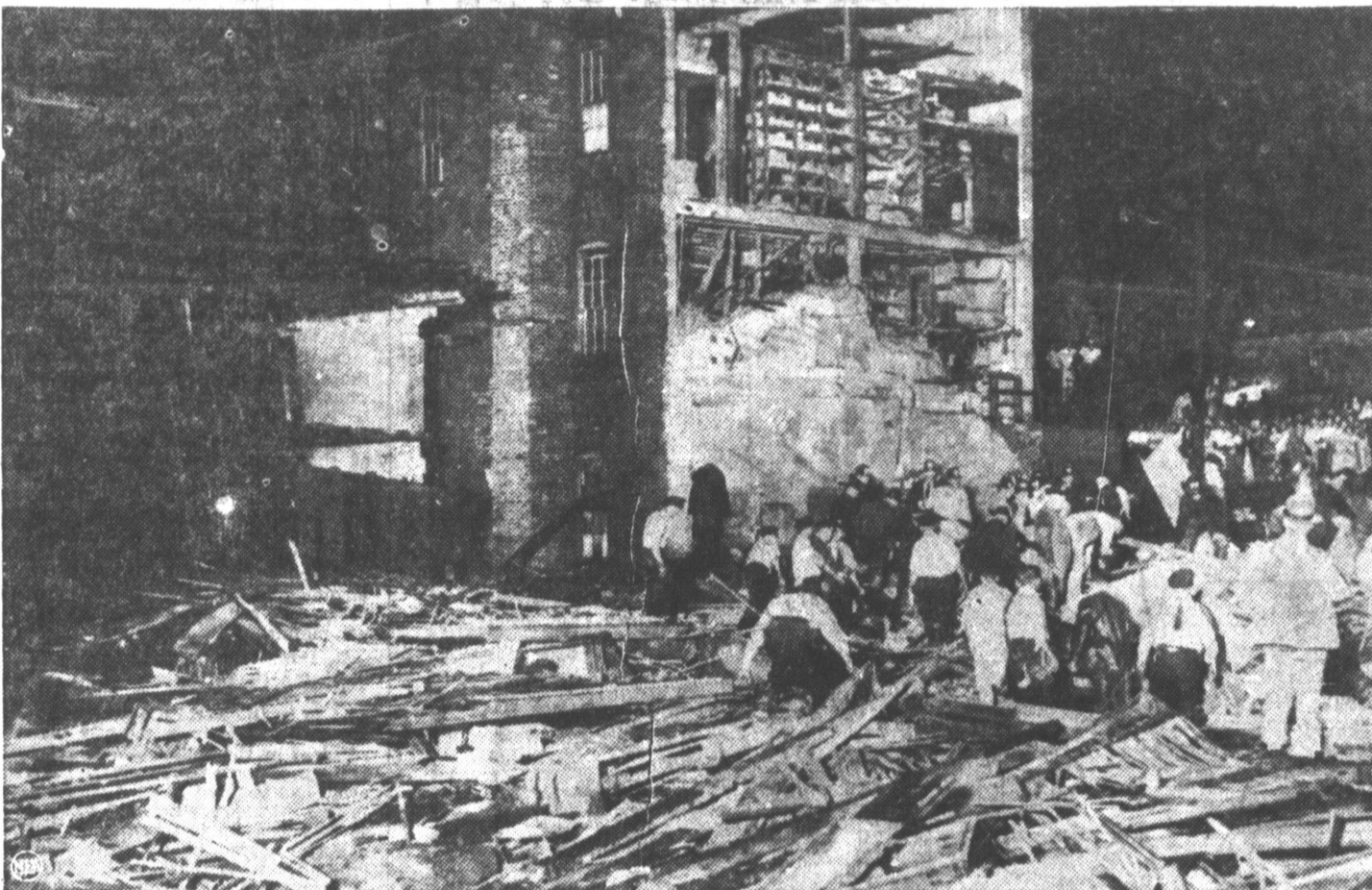
This jumbled pile of bricks, timbers, splintered walls and twisted pipes formed the tragic monument for at least 19 persons who died as their home, a six-family dwelling on Staten Island, crashed to the earth during a terrific thunderstorm. Its foundations undermined by rushing flood waters, the building fell with almost no warning, ripping the wall from an adjacent building, leaving its rooms exposed as shown here. Firemen and firemen who assisted in the frantic rescue work are shown searching through the debris.
