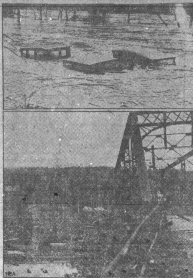
(NEA Service, New York Bureau) They weren't amphibian automobiles, and their owners had to scurry to safety when the three cars shown in the upper picture were engulfed by New England flood waters. Blow in a bridge at White River Junction, Vt., with the wreckage of another bridge piled against it—one that washed out at Hartford, Vt., a short distance up the White River, as the flood hit with full force.
