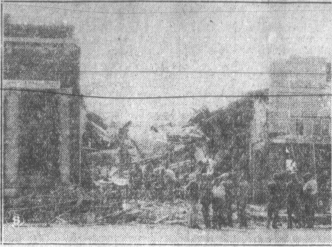
Here is the scene of the downtown gas explosion at Panhandle, Texas, which resulted in injury to four people and $50,000 damage. The blast occurred when W. H. Rogers, grocer, struck a match to look for a gas leak. Rogers, J. I. Raines, Roscoe Vance, Ed Baker, and his son, Esco Baker, were all injured, and three buildings were damaged, one being completely demolished.
