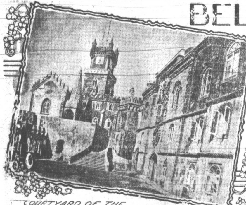
COURTYARD OF THE PALACE AT CINTRA
