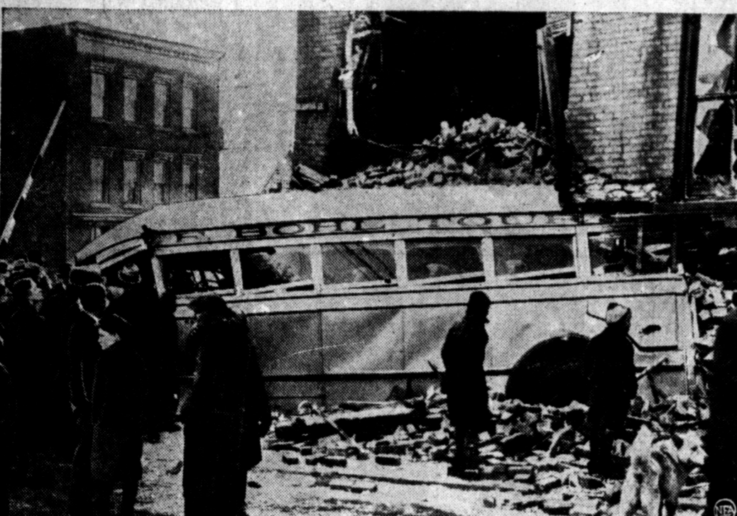
Another bus tragedy is what this picture looks like, but except for the driver, Francis Wise, who suffered lacerations of the face, the incident had a happy ending. Unable to stop on slippery pavement, the passengerless vehicle skidded onto the railroad tracks at Cobles, N. Y., and was crashed into the adjacent brick building by a train. A baby was tossed from its crib in the house but was uninjured.
