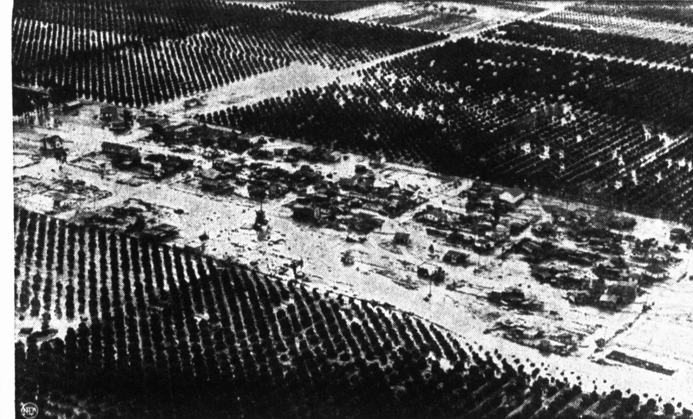
That flood water is no respecter of orange groves is shown by the picture above, taken from an airplane as unprecedented rains brought high waters that inundated the Los Angeles area, taking scores of lives and causing millions of dollars in property damage.
