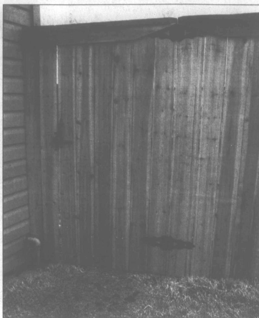
Pampa News photo by Katherine Flanary An example of a six-foot tall cedar fence that has been capped, which is an option that Cox Fencing offers. Cedar is not as common as spruce, but just as popular.
