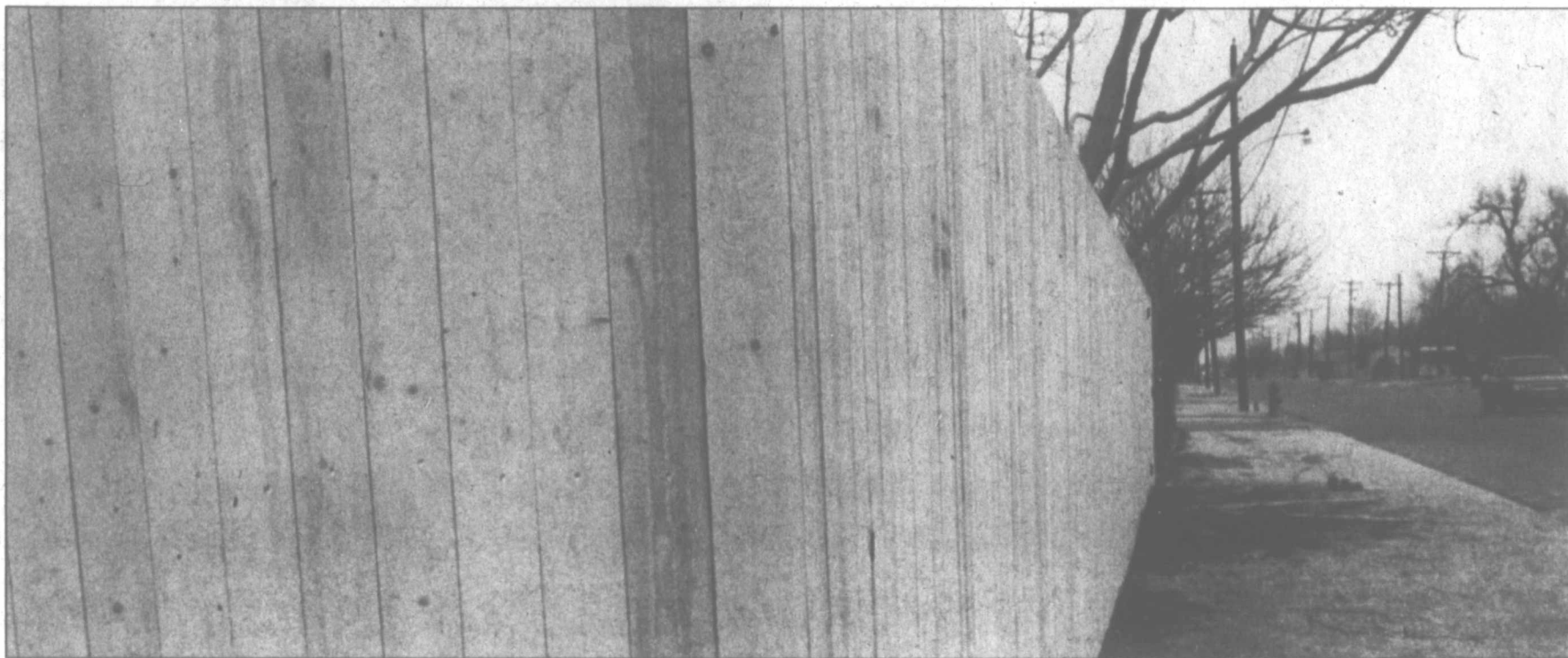
TOP: Jason Bagwell, an employee of Cox Fencing, works on the spruce fence's gate. This spruce fence is six feet tall. BOTTOM: A standard spruce fence that has been finished. This particular spruce fence is six feet tall. Spruce is the most common form of wood used when building a fence.
