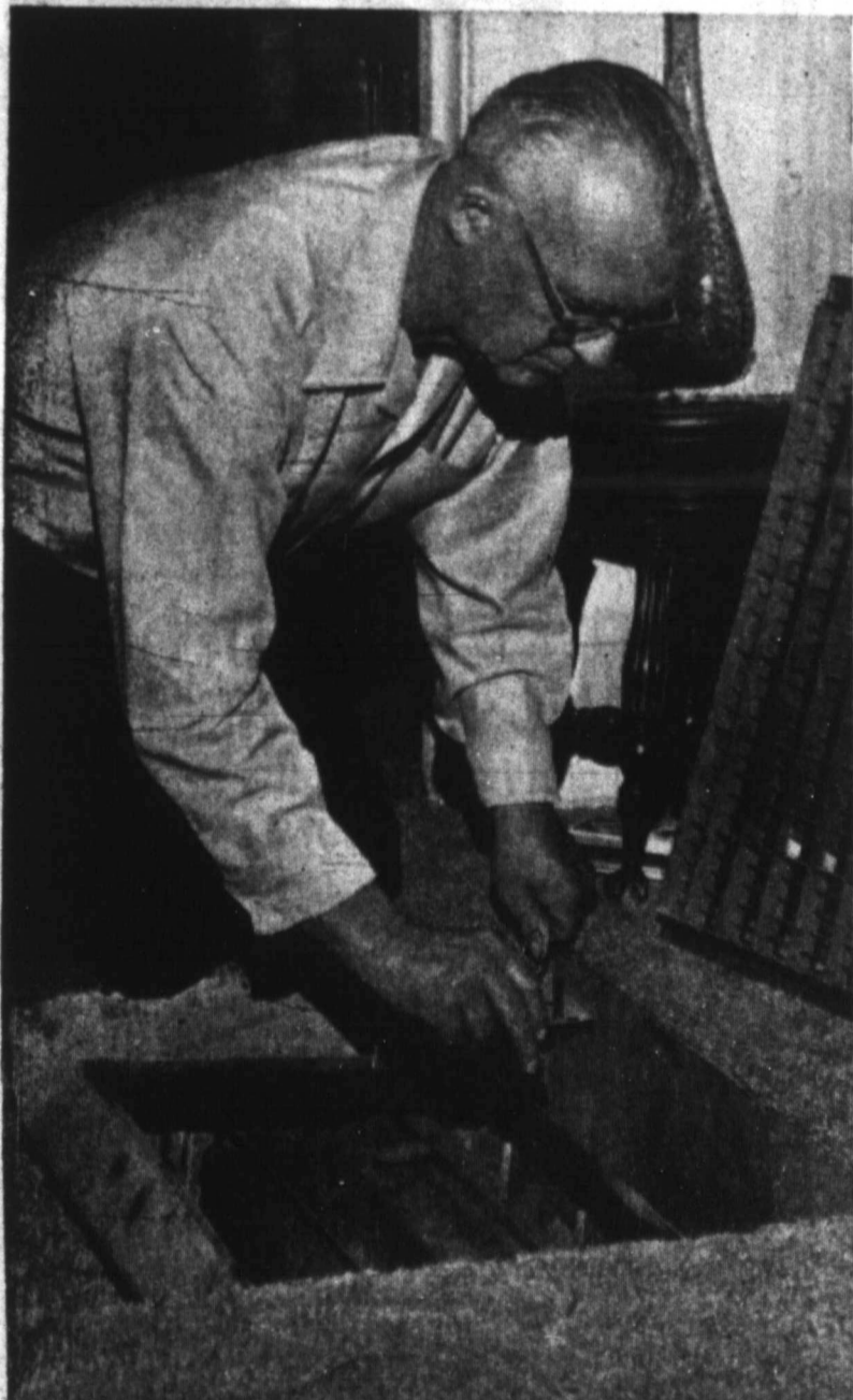
PREPARING FOR the coming winter months, Spencer Hearn, 600 N. Somerville, checks and cleans his gas floor furnace. The floor furnace, susceptible to more dust and dirt than a wall furnace needs to thoroughly inspected to prevent it from being a possible cause of fire.
