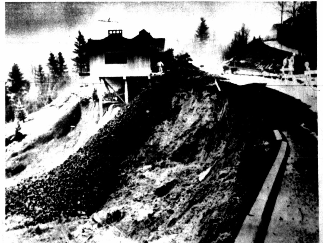
THE PERRY COLEMAN home in Gresham, Ore., perches very close to disaster after a mudslide swept out half of the street and slid down a steep
