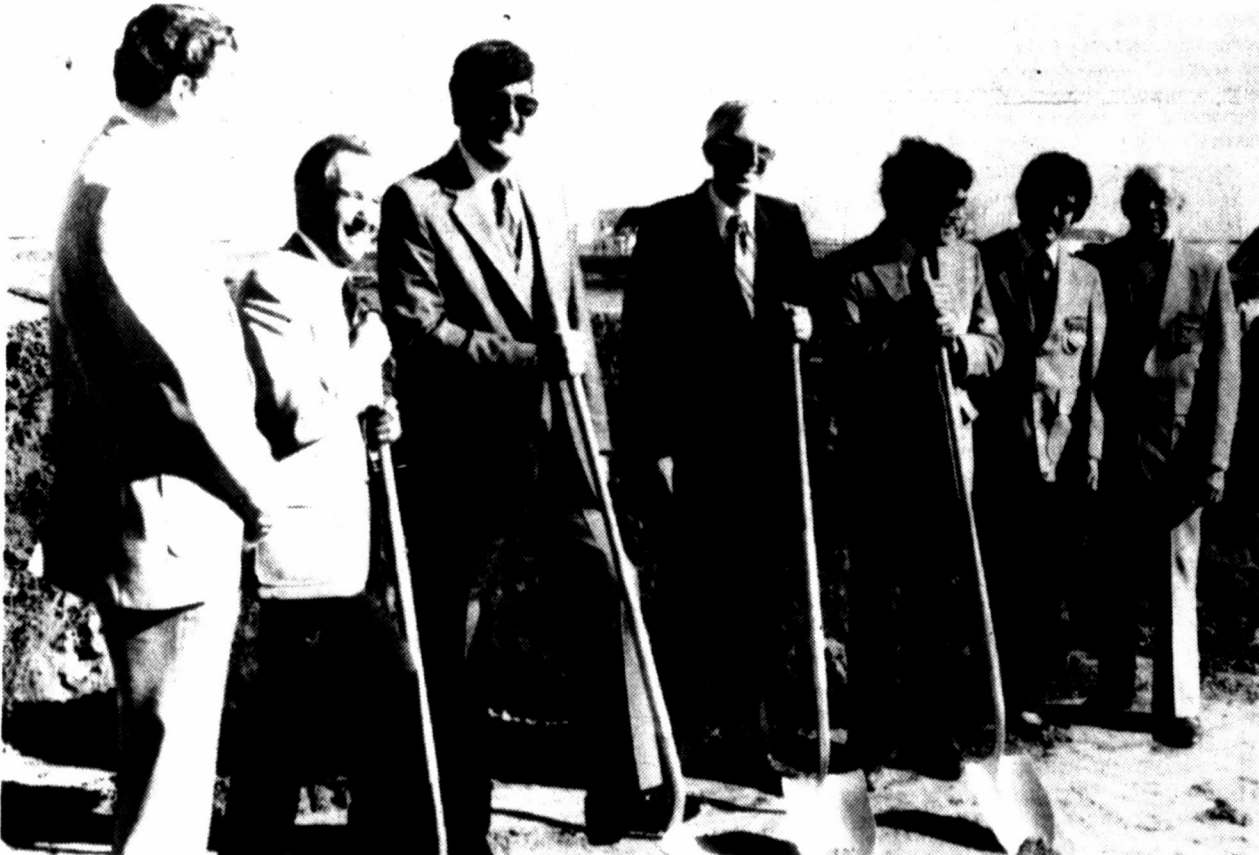
PAMPA AND SCHLUMBERGER OFFICIALS turned out Thursday to "turn the turf" for construction of a new $350,000 building for Schlumberger Well Services on West Kentucky west of Price Road. Construction of the 50- by 220-foot building is to begin immediately with Tusha Builders of Odessa as contractor. District Manager Stan Harris said company officials hope the building is completed by July or August. He said the building
