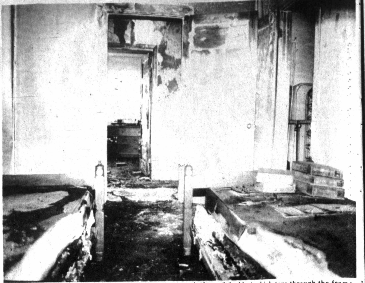
DESTRUCTION FROM FIRE EXPLOSION can be seen in this photograph of one of the bedrooms of a house burned in an early morning fire Saturday. Wallpaper and paint peeled from their surfaces in
