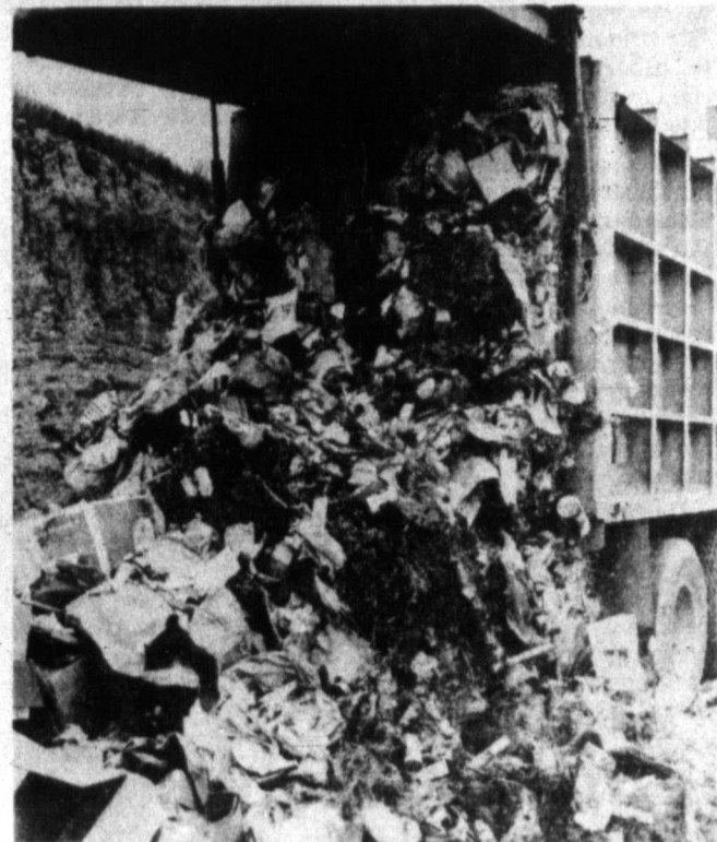
trash trucks unloads its cargo in one of the landfill trenches at the grounds. After enough garbage (the city collects an average amount of 60 tons a day) has been placed in the trench, the compactor will roll over the trash, spread it evenly and pack it down in the trench.
