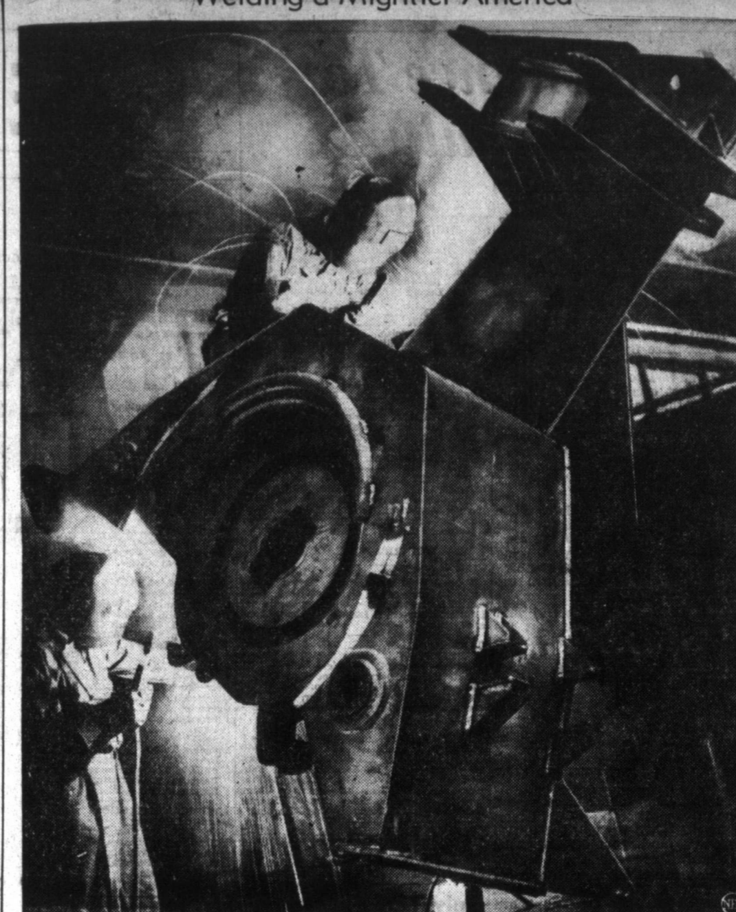
Strikingly symbolic of rearming America is this picture of welders at work on mount for a new 155-mm. gun in the Pettibone-Mulliken plant in Chicago. First mount comes off assembly line this month with production increasing steadily thereafter.
