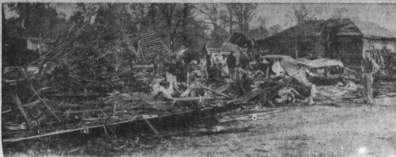
ARKANSAS TORNADOES CAUSE GREAT PROPERTY DAMAGE—Wreckage of homes
