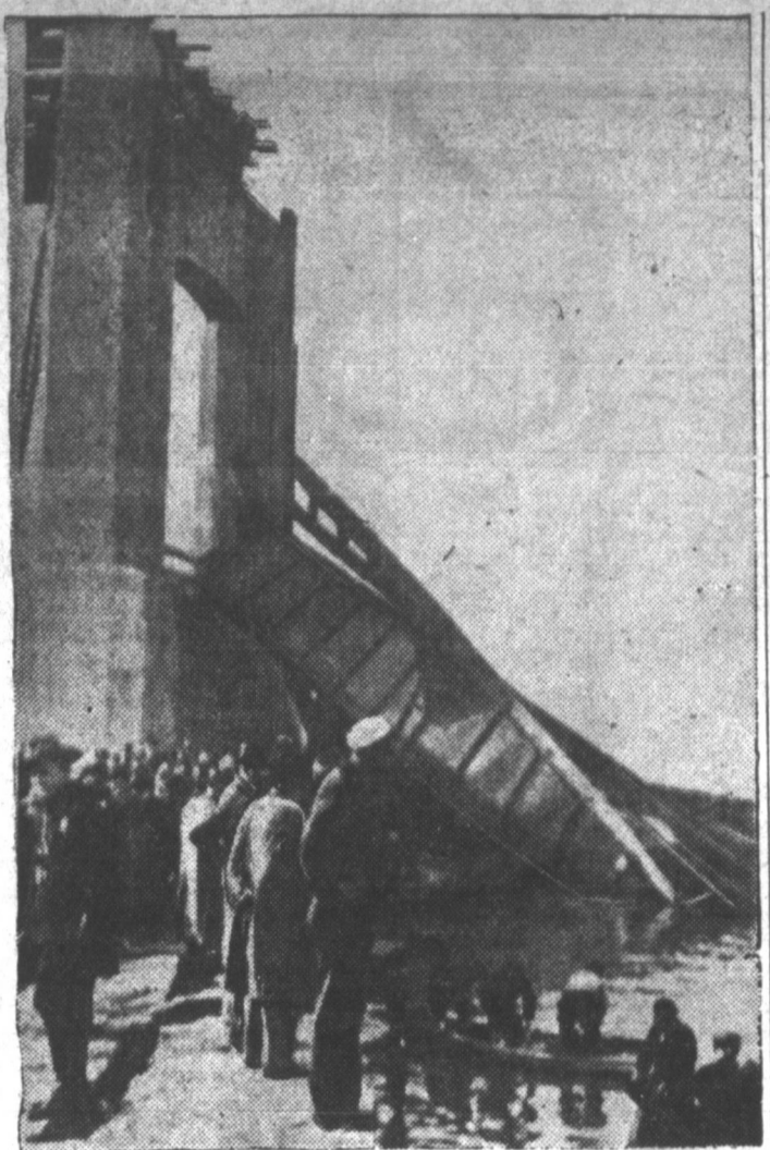
EIGHT DEAD, SEVEN MISSING IN BRIDGE COLLAPSE —Disaster, in the shape of twisting, tearing girders, struck at Hartford, Conn., when half of the water span of the new $1,500,000 Connecticut river bridge collapsed as the final link was being set into place. Workmen, including W. James Ward, supervisor and builder of the Golden Gate bridge, were plumed 8 feet amid crashing beams into the water.
