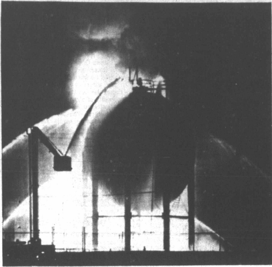
REFINERY BURNS. Firemen at the Texaco refinery in Lawrenceville, Ill., attempt to cool a 144,000-gallon propane tank early today after a fire broke out Wednesday. An estimated 1,000 residents near the blaze were evacuated. No one was reported injured at the refinery 225 miles south of Chicago on the Indiana border. Firemen at the scene estimated the fire fed from the tank would burn for 36 hours.
