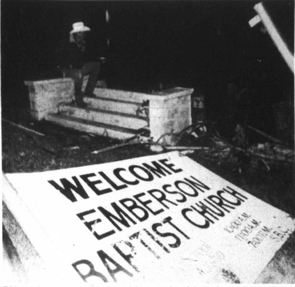
TORNADO DAMAGE. Detective John Williams of the Lamar County Sheriff's Department sits on the steps of all that remains of the Emberson Baptist Church in the northeast Texas community after it was hit by a tornado.
