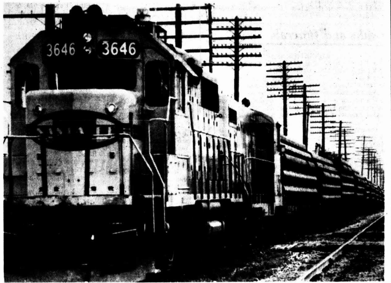
ONE OF THE FIRST TRAIN LOADS of pipe for use by the new Irish Pipe Coating Company arrived Monday morning for the plant which is located on Highway 60 on property purchased from the Packerland Packing Plant. Huge forklifts will lift the pipe from the railcars and thus save handling costs and time. The Pampa plant is one of five permanent plant locations in Louisiana, and Texas. Staff Photo
