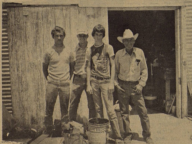
Brad Smith, Ted Johnson, Tim Taylor, and Mr. Babe Underwood have been busy repairing the roof.
