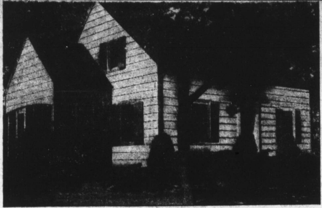
Long popular for modernization and remodeling, asbestos-cement siding shingles have come into their own as an exterior finish for new homes. How well this type of siding, developed within the past two decades, harmonizes with traditional American architecture is evidenced in the home pictured above. Asbestos siding, in addition to its unique attractiveness, has the advantage of being fire-safe and practically free from maintenance expense. The roof is covered with a companion material, asbestos roofing shingles.
