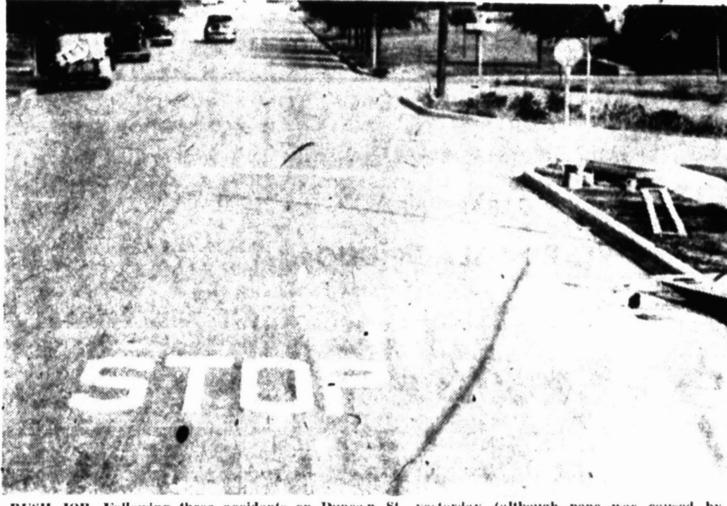
RUSH JOB —Following three accidents on Duncan St. yesterday (although none was caused by speeding city workers were painting and erecting stop signs on Duncan and Louisiana (shown above) and Duncan and Harvester Streets today. The letters "STOP" are patented as a warning. A new metal signpost can be seen in the right background. (News Photo and Engraving).
