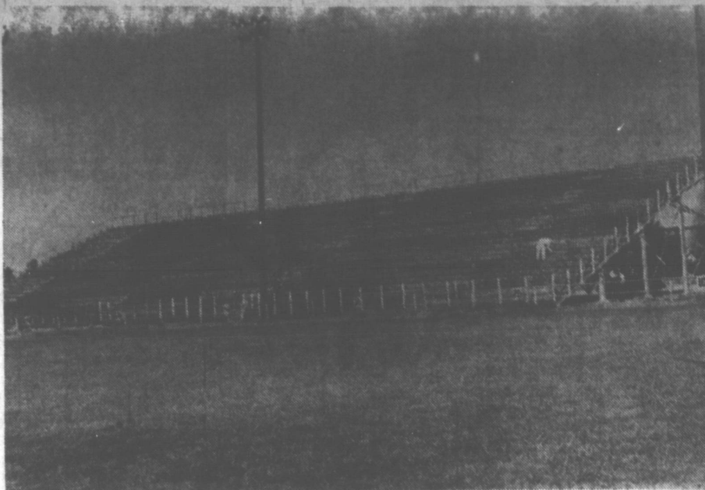
BRAND NEW—Above are shown the newly-completed stands at Harvester Park, stretching from the 20 to the 30. The stands, replacing an older structure, blown down last summer, will seat 2,520 football fans and bring the total seating capacity for the field to 5,158. (News Photo and Engraving)
