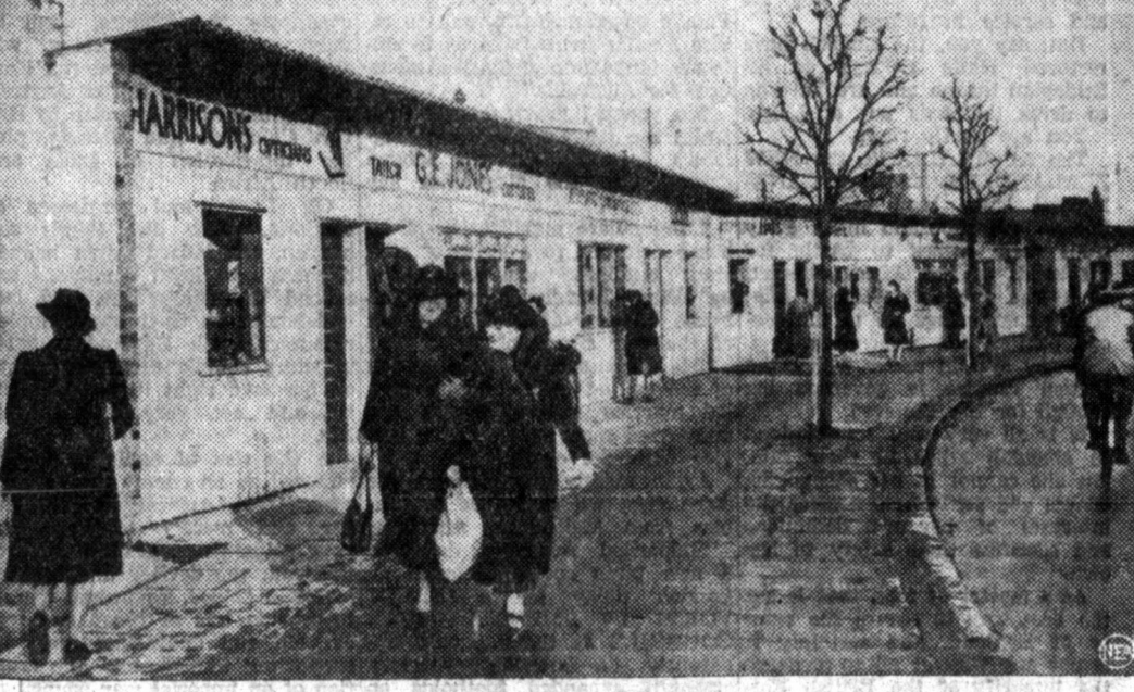
BUT COVENTRY TODAY is marching ahead toward victory. Where homes were wiped out, better homes safer from bombs have been built. Emergency shops, like those above, neat and simple, have gone up where the bombers blasted the city's business districts.
