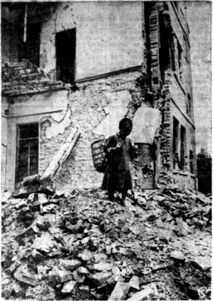
The very young help with rebuilding Chungking. This lad is looking for something worth salvaging.
