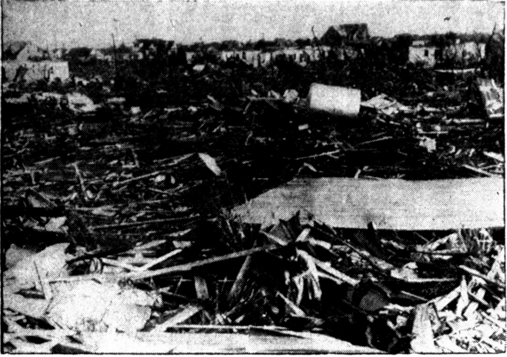
HOMES REDUCED TO SPLINTERS BY TEXAS TORNADO—Where homes once stood only splintered debris was left in this scene near the center of the residential district of Crowell, Tex., after a disastrous tornado.
