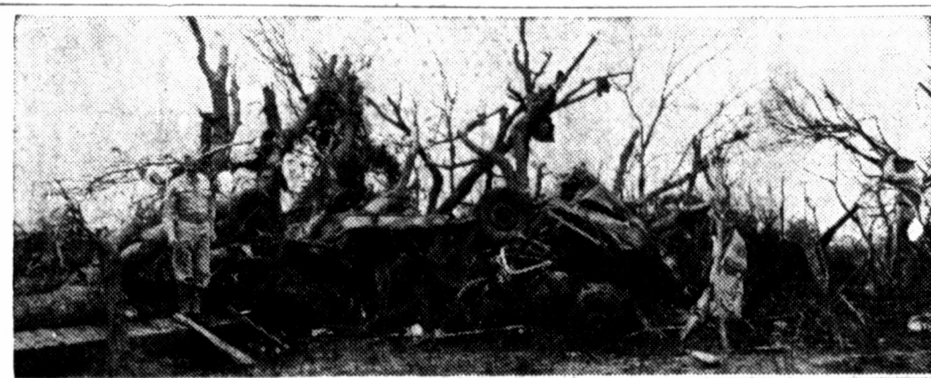
30 DEAD IN OKLAHOMA CITY TORNADO—Latest reports indicate that 30 persons were killed and more than 25 injured in the tornado that swept through a residential
