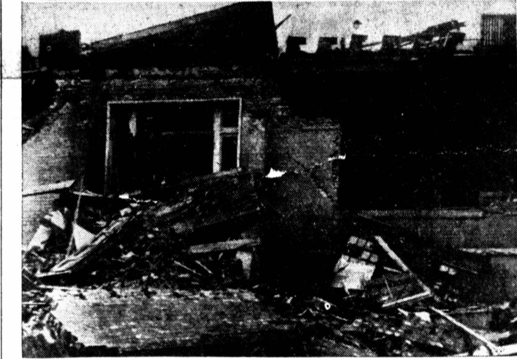
With 25 persons known dead, rescue workers dug into the debris of shattered homes and business buildings at Berryville. Ark., searching for other persons believed killed when a tornado struck this small town. At the top is shown a general view of Berryville after the tornado struck and at the bottom the remains of a schoolhouse. (NEA TELEPHOTO)
