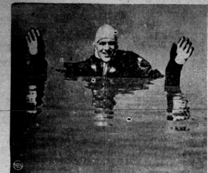
War-time life-saving outfit, worn over regular uniform, keeps torpedoes warm and dry. Buoyant suit, developed by Goodrich, has weighted boots which keep wearer upright in water.
