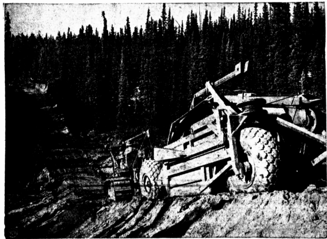
This mighty machine of peace-time, a tractor-drawn carry-all, helps build a wartime highway to Alaska through the forested Canadian wilderness. U. S. Army engineers constructing the road use this machine to move tons of earth from one section of the route to a fill.
