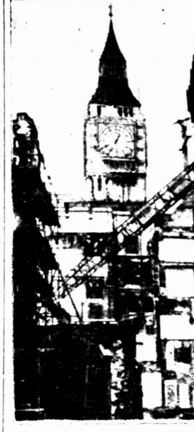
Work of cleaning ruins of blitzed House of Commons, London, England, now is completed and site stands ready for rebuilding.
