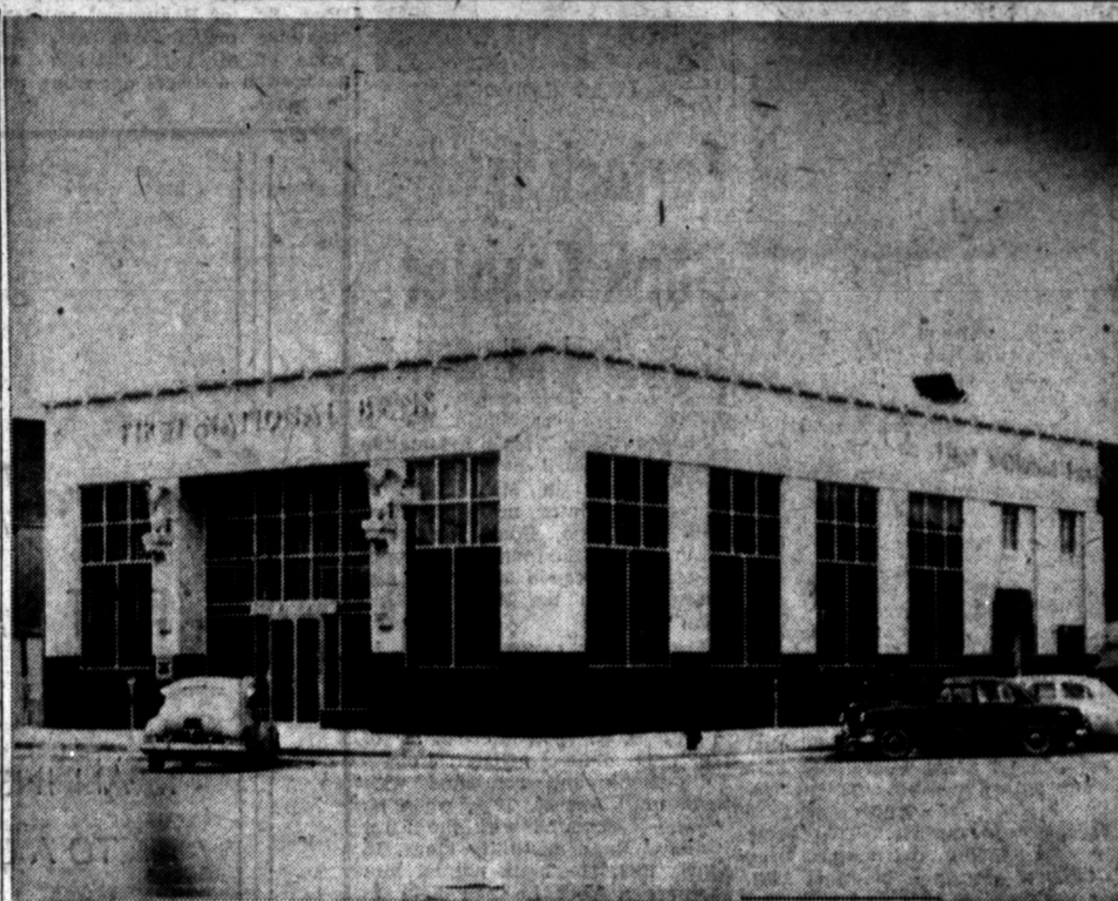
READY FOR BUSINESS —Open house will be held in the new First National Bank building tomorrow and the wheels will start to turning for good Monday. Started in early April last year, the building is now finished. The letters above the large glass doors are of steel and stand out from brick wall. The national eagle on each side of the doors depicts the strength of the bank. C. S. Lambie is the general contractor. The windows are of functional lighting value. (News Photo and Engraving)
