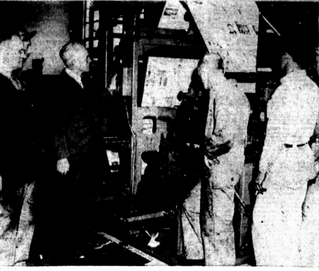
FIRST RUN—Once again, The Pampa Daily News comes off its own press, this time in its new home at S. Somerville and Atchison. Pressmen and mechanics who helped install it in the new building took on...
