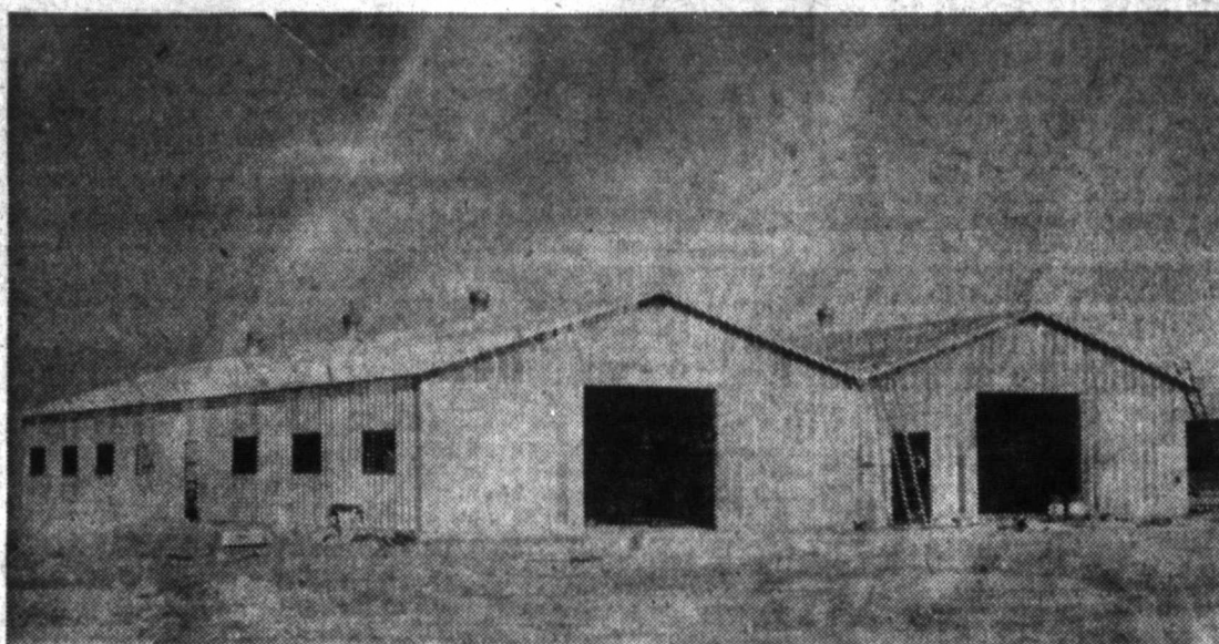
HBA BUILDING —The 1951 Top o' Texas Hereford Breeders Assn. show and sale, to be held this coming Monday and Tuesday, will be conducted in this new 6136-foot building at Recreation Park. The building is an all-steel Butler creation and will easily take care of all entries in the show. It was erected by the Link Tschudy company of Amarillo and was completed a short time ago. Members of the HBA bought and paid for the building out of their own pockets and with the aid of interested outsiders. (News Photo and Engraving)
