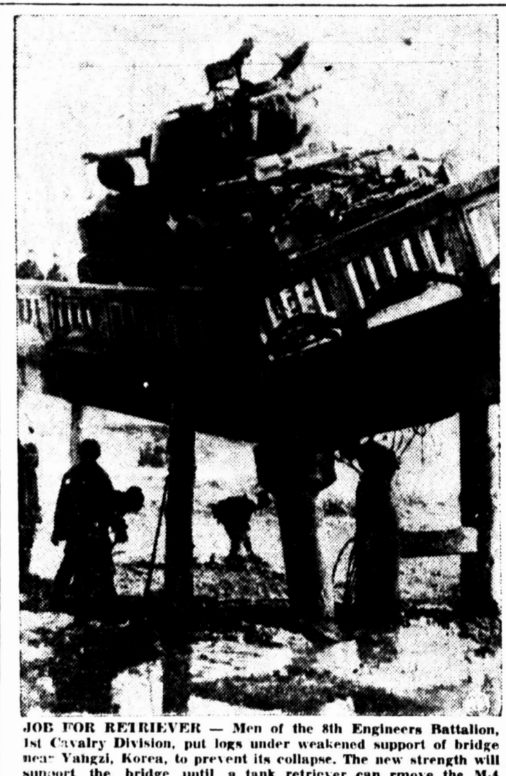
JOB FOR RETRIEVER — Men of the 8th Engineers Battalion, 1st Cavalry Division, put logs under weakened support of bridge near Yangju, Korea, to prevent its collapse. The new strength will support the bridge until a tank retriever can remove the M4 which is stranded. (NEA Telephoto)
