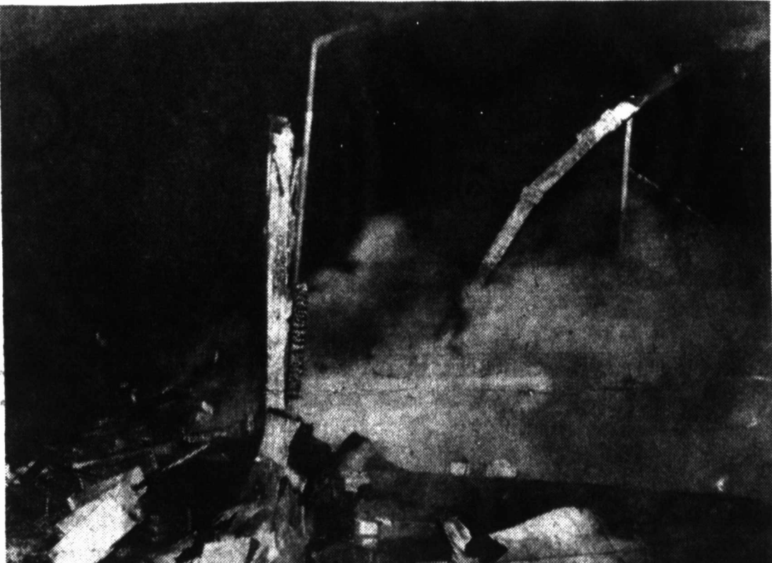
RUINED BY FLAMES — Pampa's National Guard armory at Recreation park was nothing but a smoldering ruin this morning after flames from an undetermined origin completely destroyed it and its contents. Looking south from the north end of the building, fireman can be seen still pouring water on the last embers as steam and some smoke roll southward. It was 9:30 a. m. before debris was cool enough for firemen and guardsmen to remove the remains of equipment from the structure. (News Photo)
