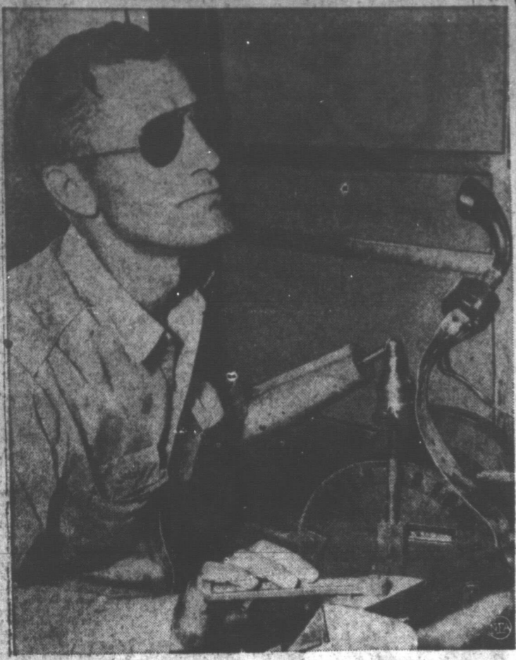
ATTACHED TO HIS JOB —Literally bolted to his job by a steel ball bearing wrist is Ralph Olson, cableway operator at Hungry Horse, Mont. Olson himself designed the special steel joint that connects his artificial left arm to the cableway speed control.
