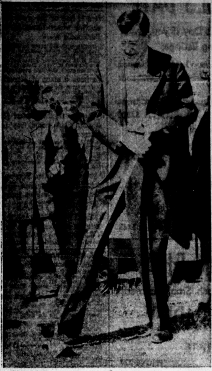
GROUND-BREAKING —N. A. Cobb, 1104 Christine, turns the first shovelful of dirt for the foundation of the new Church of Christ to be constructed at Harvester and Mary Ellen. Ceremonies were held Saturday morning for the groundbreaking. Cobb also broke ground for the old church on Francis Avenue 25 years ago. Standing near him is Mrs. Mable Kennedy, who was present when the old building was started. The new church will seat 600 persons and will cost approximately $160,000. (News Photo)
