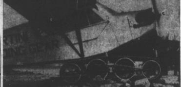
PLANE MAKES TRACKS—This caterpillar track landing gear for a light plane was developed by Count Giovanni Bonmartini in Rome, Italy. He says the tracks enable the plane to land on any type of ground, with or without regular landing facilities. (NEA-Acme photo-by Staff Ehotographer Albert Blasetti.)
