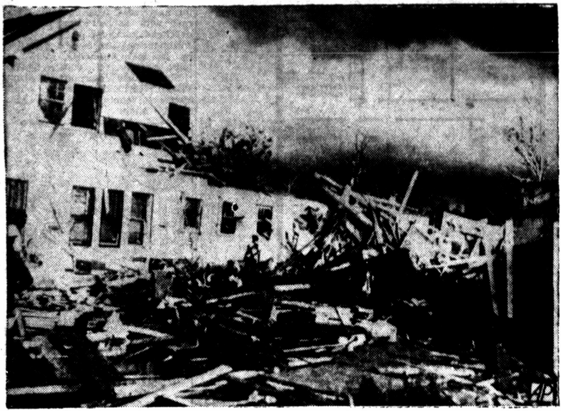
TORNADO PATH—The two-story house (above) fared better than the building next to it in a tornado that swept through the north Texas town of Olney. The twister literally wiped out a two-hundred-yard section of the town. Two were killed and about 100 injured. (AP Wirephoto)
