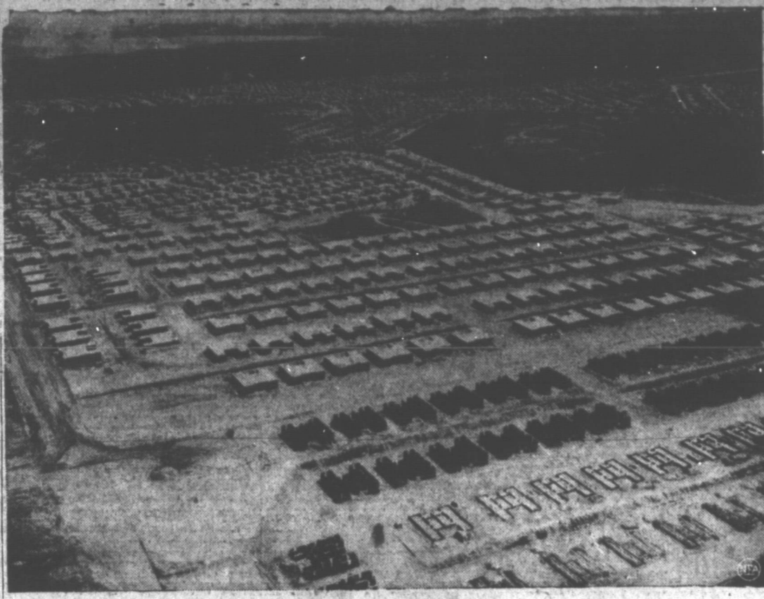
HOUSING BOOM —Construction is now the third largest industry ($75,000,000 in 1950) in Puerto Rico's booming economy. One contractor has a 10,000-man payroll, spends $17,000,000 for labor wages. Typical of the little island's great housing projects is this vast development at Puerto Nuevo. Originally started with about 5000 small houses, 3500 duplex bungalows (foreground) are being added. They will provide homes for 7000 families.
