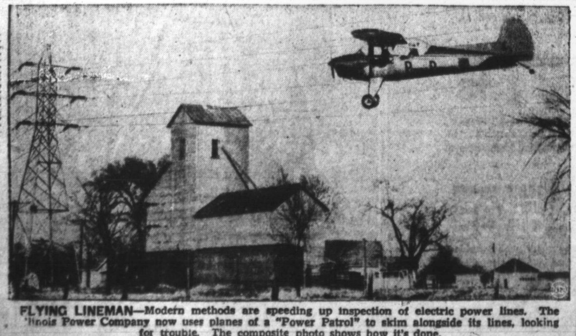
FLYING LINEMAN—Modern methods are speeding up inspection of electric power lines. The Illinois Power Company now uses planes of a "Power Patrol" to skin alongside its lines, looking for trouble. The composite photo shows how it's done.
