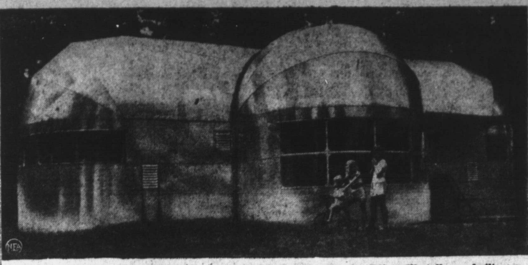
ON HIS METAL —This aluminum alloy home, designed by Thomas Edison Westall, was built near Marion, N. C. Said to be dustproof because all air entering the house is filtered by air-conditioning units, it has cornerless rooms, curved windows of transparent plastic and floor space equivalent to that of the average five-room, conventional house.
